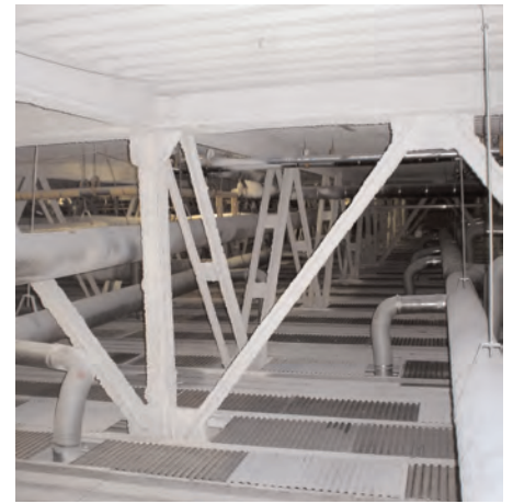
Completed Encasement system after application of the FiberTech F-51 sealer coat
