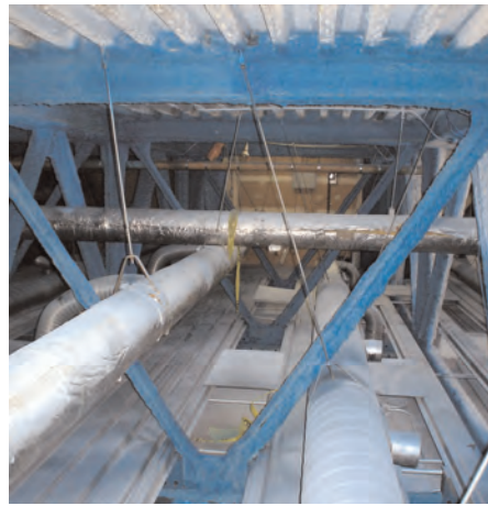
Primed Fireproofing using Fibertech F-50 penetrating primer
